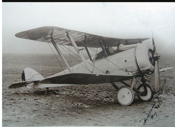
BRITISH PHOTO OF A PROTOTYPE SE5 A4562 AT ST. OMER THE SECOND OF THREE PROTOTYPES. APPEARS TO HAVE AN EXPERIMENTAL ARRANGEMENT REGARDING THE ALDIS LIGHT AND THE COCKPIT WIND SCREEN ON THE 28 th JANUARY 1917 ON A TEST FLIGHT FLYING TOWARDS FARNBOROUGH AT A 1000FT THE PORTWING BROKE UP A CRASHED KILLING FRANK GOODDEN.
