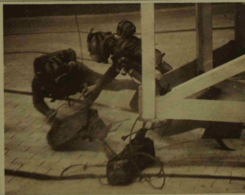
"FROG-MEN" PLACING DEMOLITION CHARGES AT CAREFULLY-SELECTED POINTS OF A GERMAN UNDERWATER OBSTRUCTION REPRODUCED FOR PRACTICE PURPOSES: THEIR SKILL RESULTED IN THE WRECKING OF 3000 OF THESE OBSTACLES OFF THE D-DAY BEACHES.
